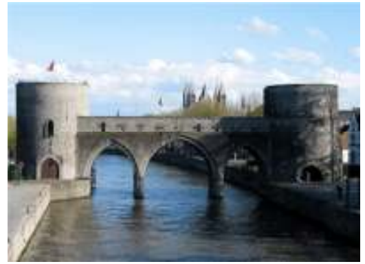
"Pont des Trous" bridge
